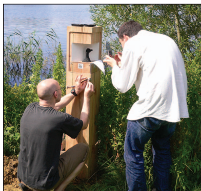
FIGURE 1 Installing a post by the lake shore.
